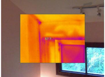
**IR000134.IS2** 5/4/2011 10:52:00 AM Poorly installed insulation allows air movement inside walls
