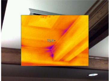
**IR000144.IS2** 5/4/2011 11:11:33 AM Air leakage around coffered ceiling trim
