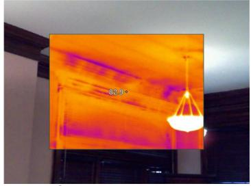
**IR000124.IS2** 5/4/2011 10:34:56 AM Air infiltration can be seen most noticeably along the top edge of the crown molding and also at other joints.
